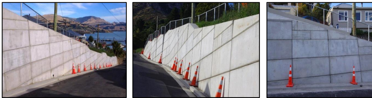
Figure 8: The completed Stone ® Strong pile supported gravity structure
