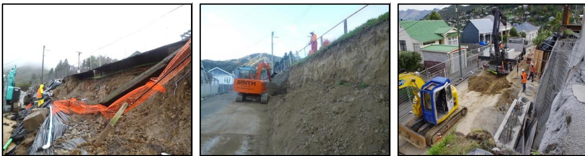
Figure 6: Reconstruction process of the collapsed wall and temporary shotcrete support
